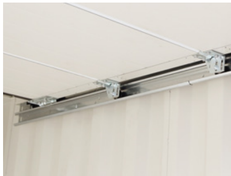
Low height from top of door to roof
